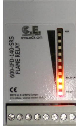
Relay will change status approx. at the 3rd led.
